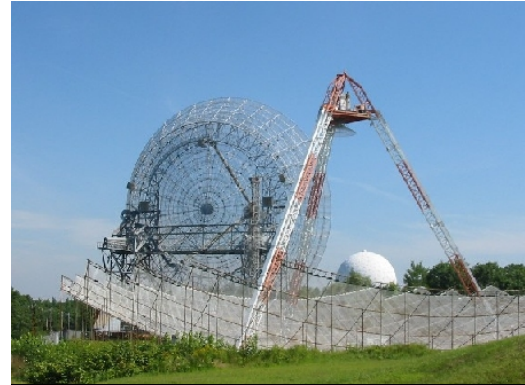
Millstone IS Radar, Westford, MA
