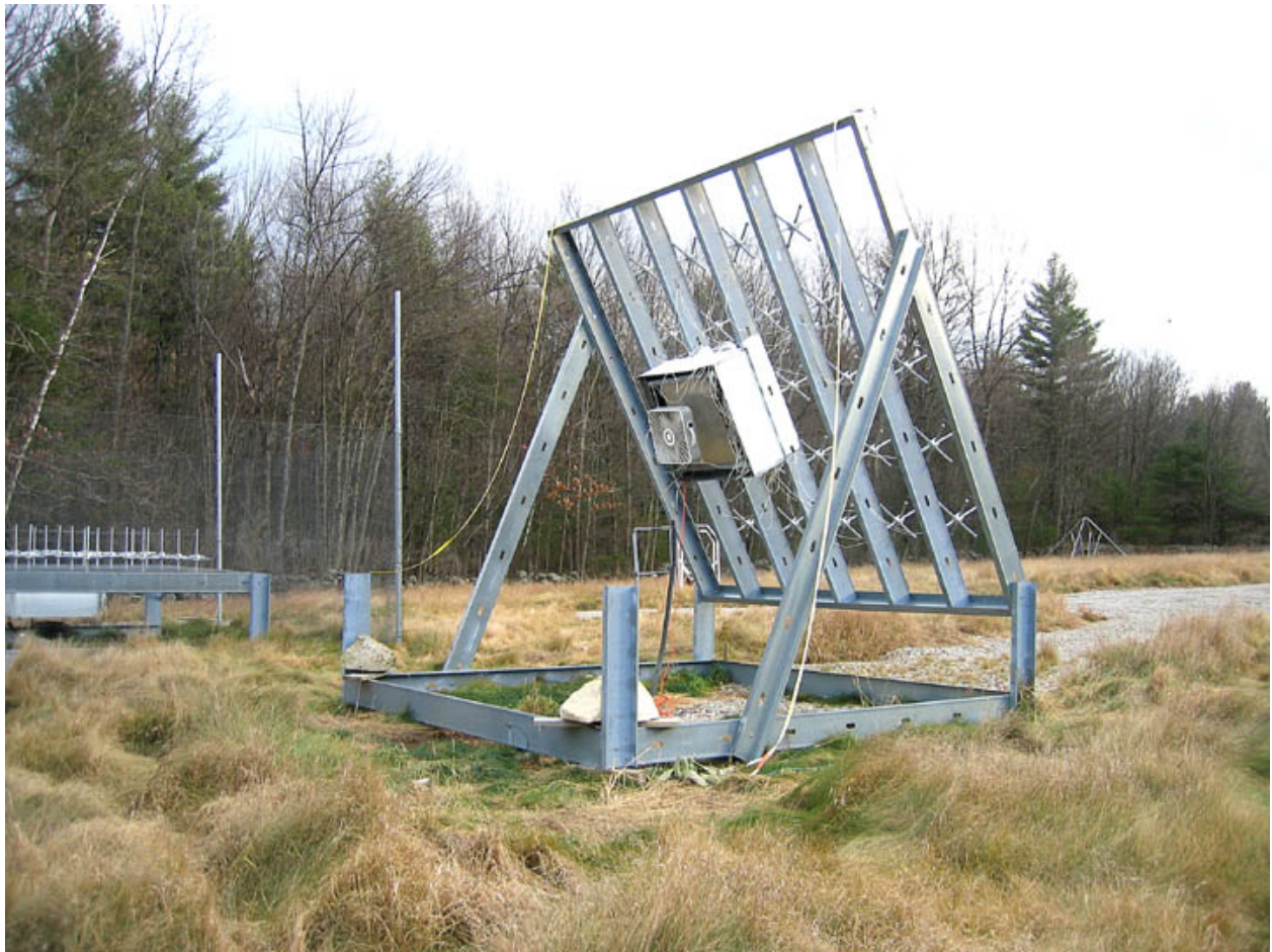
Figure 1 Station d02 tilted to point at 30 degrees elevation during test made in December 2004.
