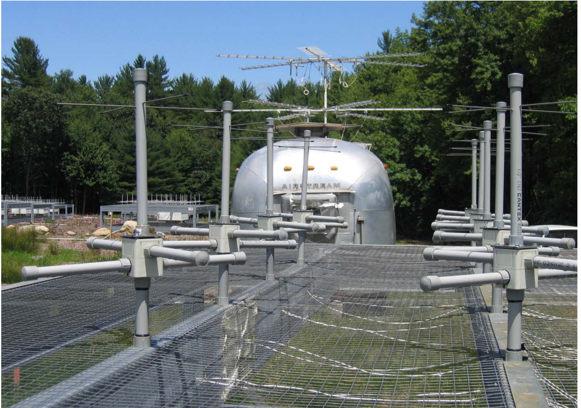
STATION D00 WITH RFI MONITOR IN BACKGROUND
