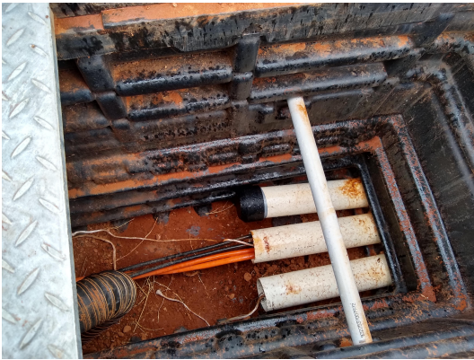
(a) Black ABS cap fitted to far end of conduit in pit.
