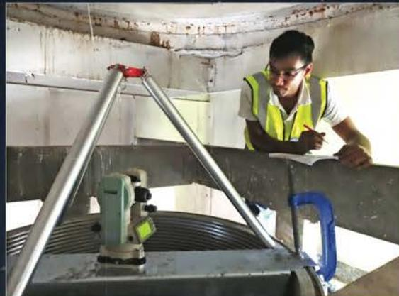
Ghana preparation – checking mirror alignment, replace feed cover and clips, pintel bearing limit switches, refurbish brakes.
