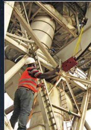
Ghana replacing shock absorbers, stow pin brackets, stow pins, limit switches.
