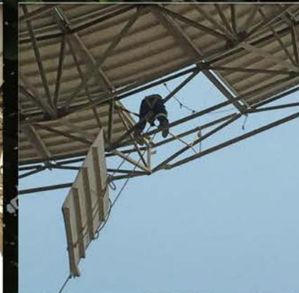
Ghana removal of damaged reflector panels for repairs.
