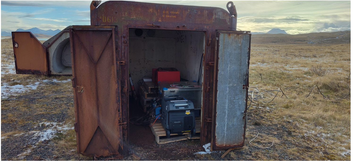
Figure 2: The electronics hut, with the generator, electronics box, batteries, and red fuel tank installed.
